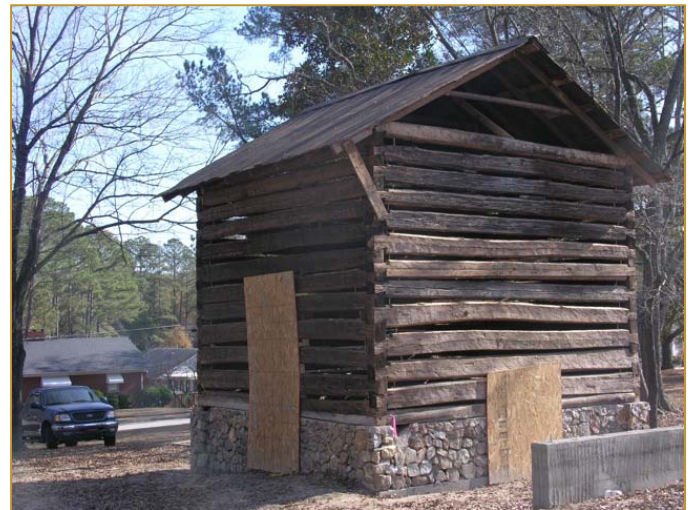
Tobacco barn stand ready for finishing touches
